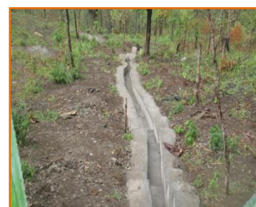
Catch water drain
