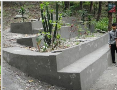
Cement Rubble Masonry wall
